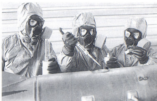
Soviet specialists remove nerve agent (diluted sarin) from a bomb during a demonstration of their mobile chemical weapon destruction system at Shikhany in October 1987. The Soviets still lack a destruction capability adequate to their huge stocks of chemical weapons.
